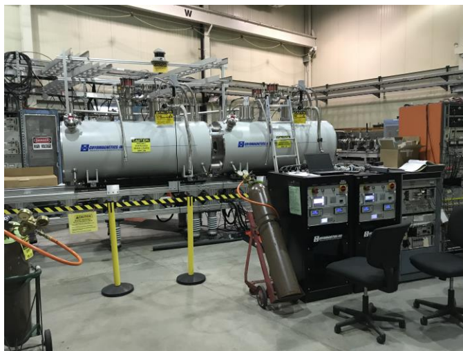
Fig. 1. Two Solenoids in the EBIS Test Area at Brookhaven National Lab.
